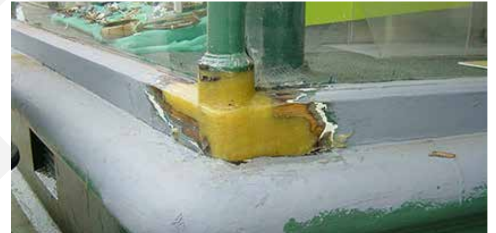
Figure 55. Resin repair to timber shopfront detail
