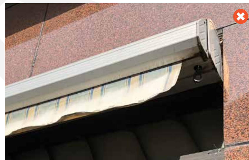
Figure 47. Blind box not well integrated with shopfront
