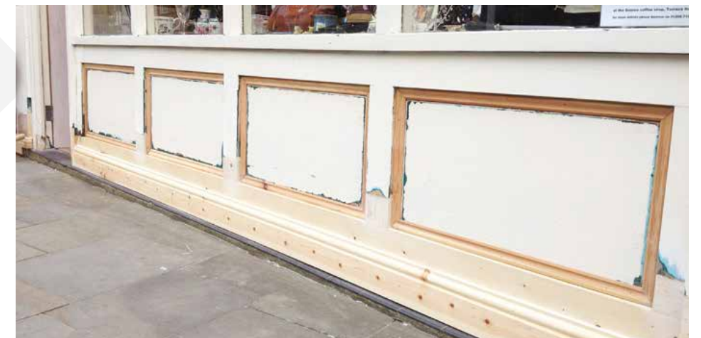
Figure 56. Timber stallriser repair
