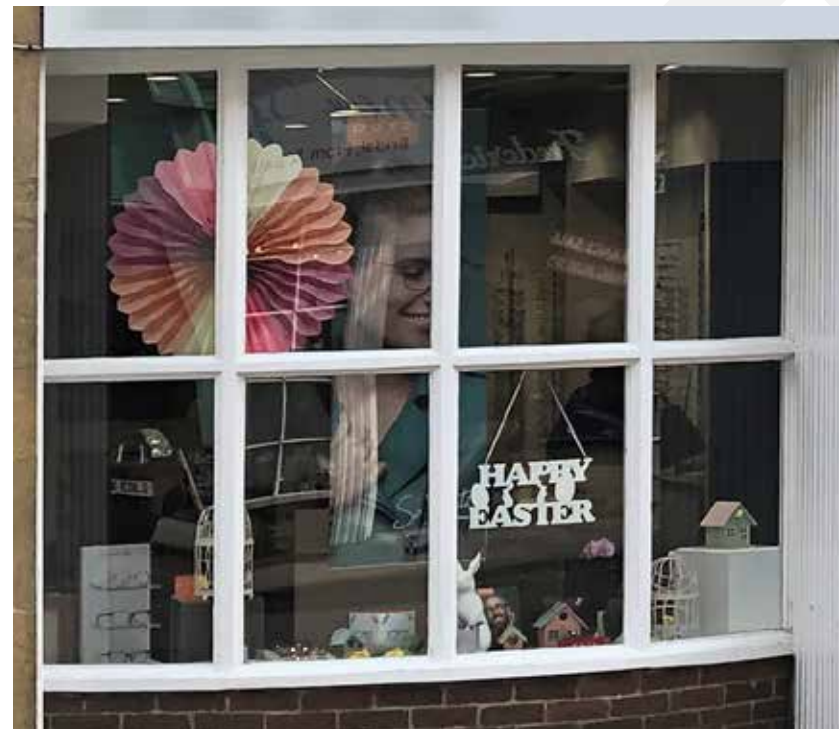
Figure 20. Timber mullions and transoms subdividing shopfront display
