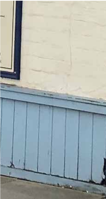
Painted brick and timber stallriser
