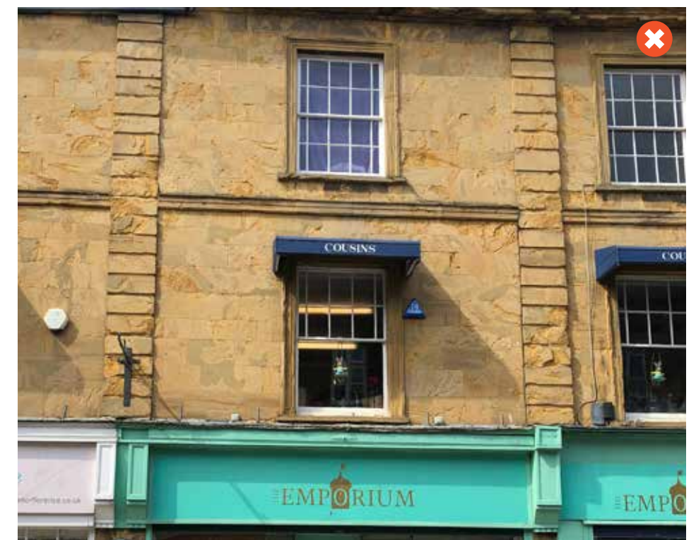
Figure 54. Alarm boxes haphazardly positioned on facade
