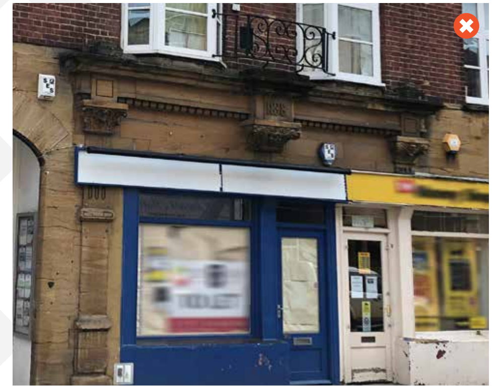
Figure 51. Alarm boxes haphazardly positioned on facade
